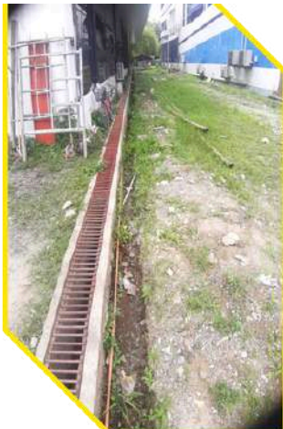
Excavation for Fiber Optics of CSU Smart Classroom
