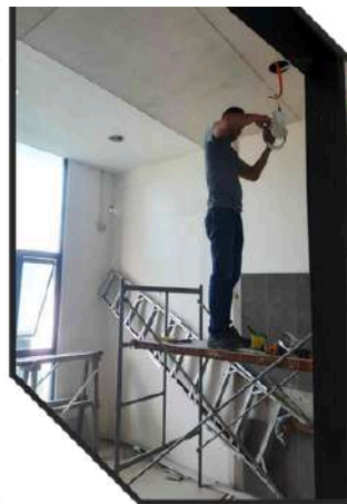
Construction of Wall Partition at Attorney's Office
