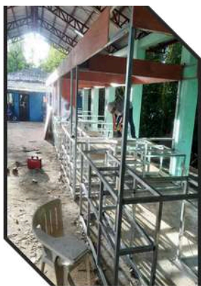
Construction of Food Stall
