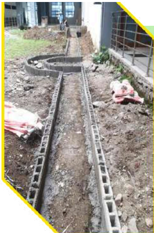
Installation of Bricks at CCIS Building
