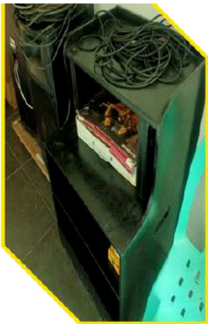
Electrical Equipment Shelves
