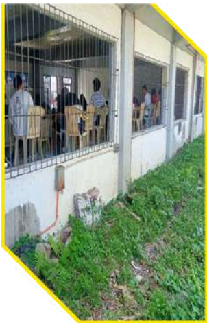
Window Grills at S&T Building
