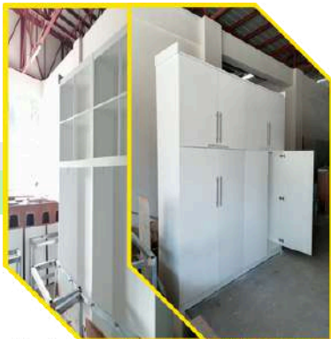
Repair of Dressing Cabinet at Executive House
