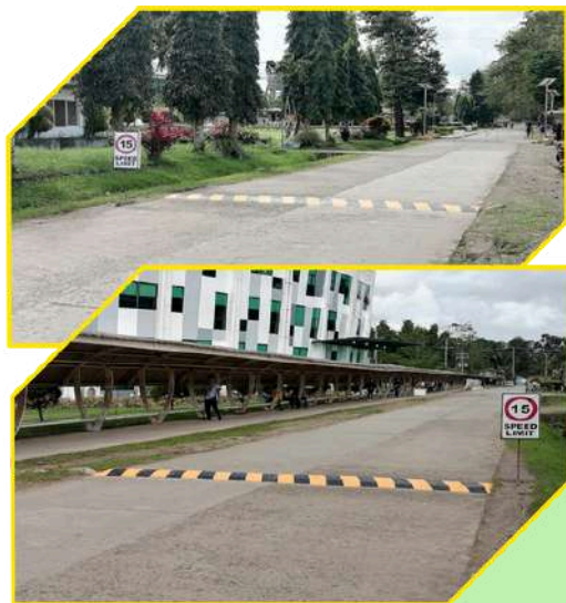
Repainting of CSU Speed Hump
