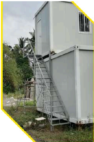
Metal Stairs at Records Office
