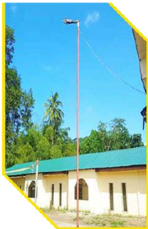
Installation of Outdoor Lamp for PE 4 at Hostel building
